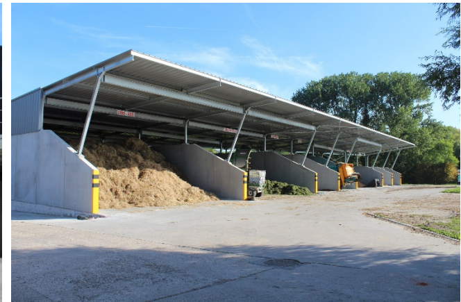
Additions to compost site (2019)
